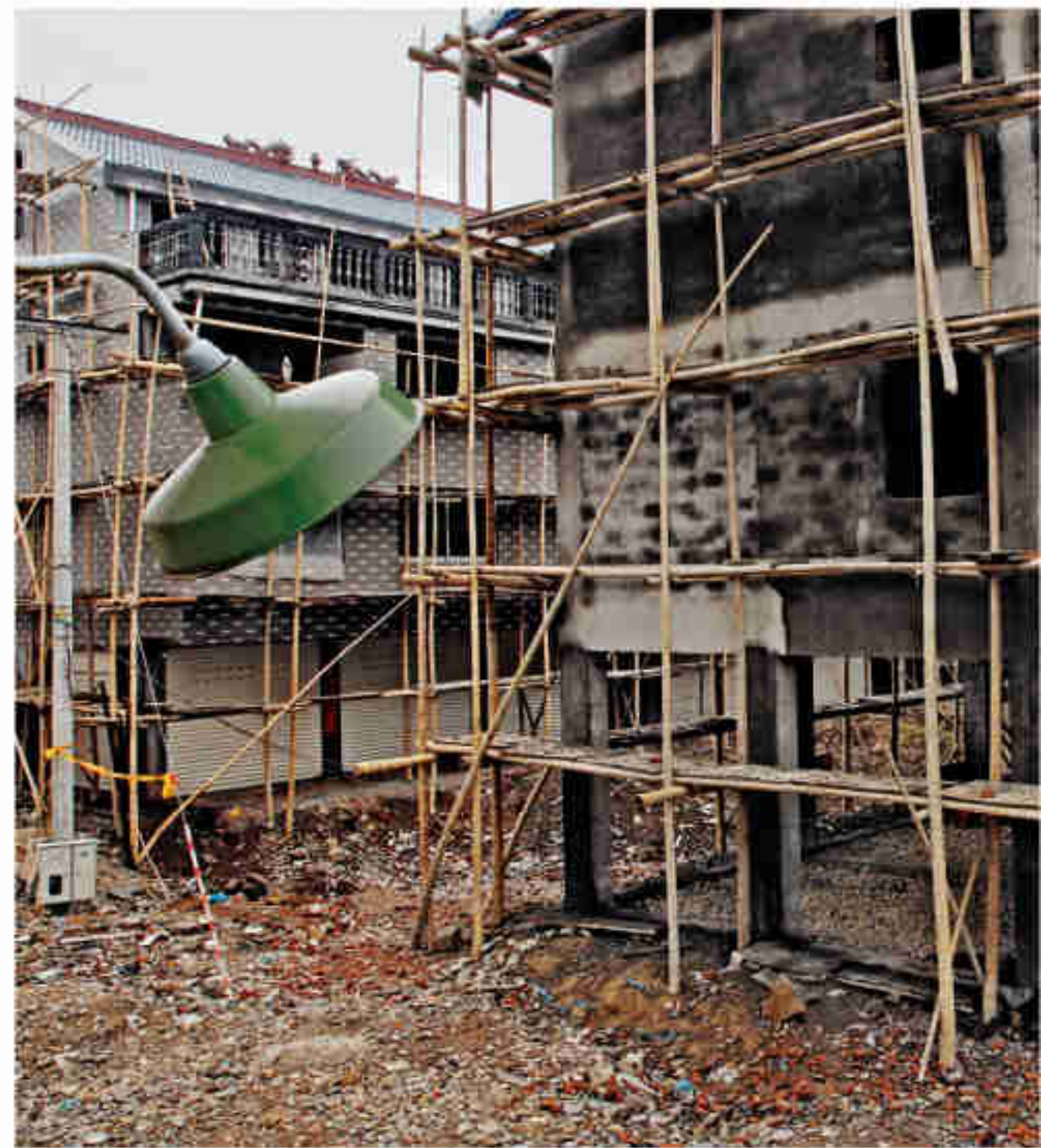
APRIL 2006: SIDING WORK
